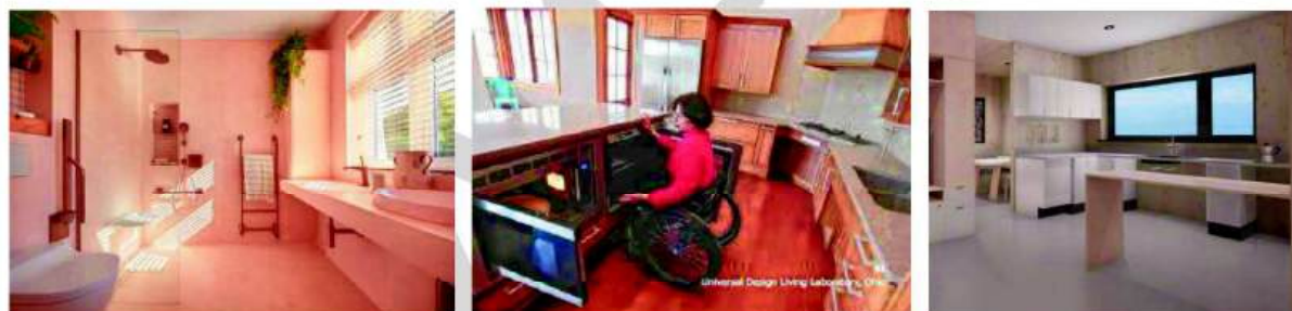
(Left) Motion spot – fully accessible bathroom. (Middle/Right) Adjustable / accessible kitchen counter tops integrated into standard design layout.
